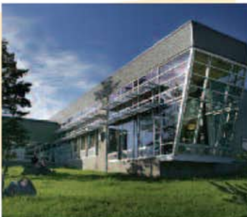
The Homer Foundation took a leadership role early in the effort to build the new Homer Public Library. Photo by: Chris Arend
